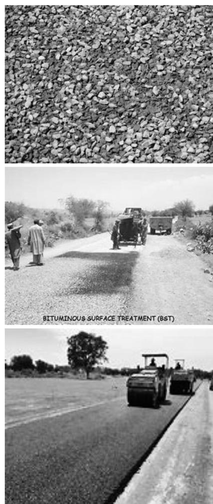
写真-2 Double Bituminous Surface Treatment(DBST)
